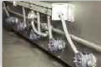
Five (5) 18 K.W. screw plug immersion heaters with stainless steel elements.
